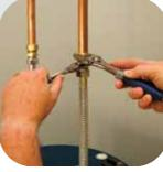
Install the hot and cold water lines. The water heater's inlet and outlet connections contain nonmetallic parts. Don't solder pipe directly to these connections. Instead, solder threaded adapters to short pieces of pipe so that soldering is done a foot or so from the water heater connections. Open the cold water supply valve and fill the tank.
