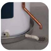
Drips from the Temperature and Pressure (T&P) Relief Valve discharge pipe usually mean you need a thermal expansion tank or your home's water pressure is too high (see Step 3). Warning: Do not plug or cap the T&P discharge pipe.
