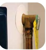
The Temperature and Pressure Relief Valve (T&P) is an important safety device. It opens to relieve pressure if the water temperature or pres- of no more than 6 inches sure is too high. Use the new T&P that came with your new water heater. Don't reuse the old T&P valve.
