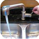
Open a hot water faucet and let the hot water run until it's cool. Then, shut off the cold water supply to the water heater. Leaving the hot water faucet open will help the tank drain.
