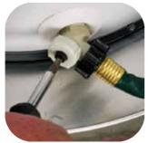
Connect a garden hose to the drain valve. Place the other end of the hose in a drain or outside (you could also use buckets). Open the water heater's drain valve. While the water heater is draining, read the Installation Instructions that came with your water heater. Disconnect the water and power lines and remove the old water heater.
