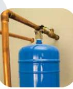
Almost all homes have check valves in the plumbing system and now need a thermal expansion tank installed near the water heater. The expansion tank is attached to the cold water inlet line. To operate properly, the expansion tank must be pressurized with air. Refer to the expansion tank's instructions for details.
