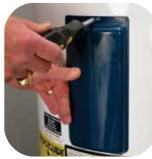
Replace the insulation, plastic protectors, and the upper and lower access panels. Replace the cover on the electrical junction box (on the top of the water heater).
