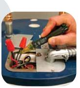
Because circuit breakers can be mismarked, always check the incoming power wires with a voltmeter or circuit tester to make sure the circuit you are working on is OFF.
